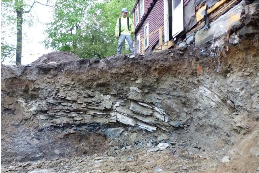
Figure 2.7. Profile of the construction excavations for the new ell cellar showing the shallowness of the bedrock around the house.
